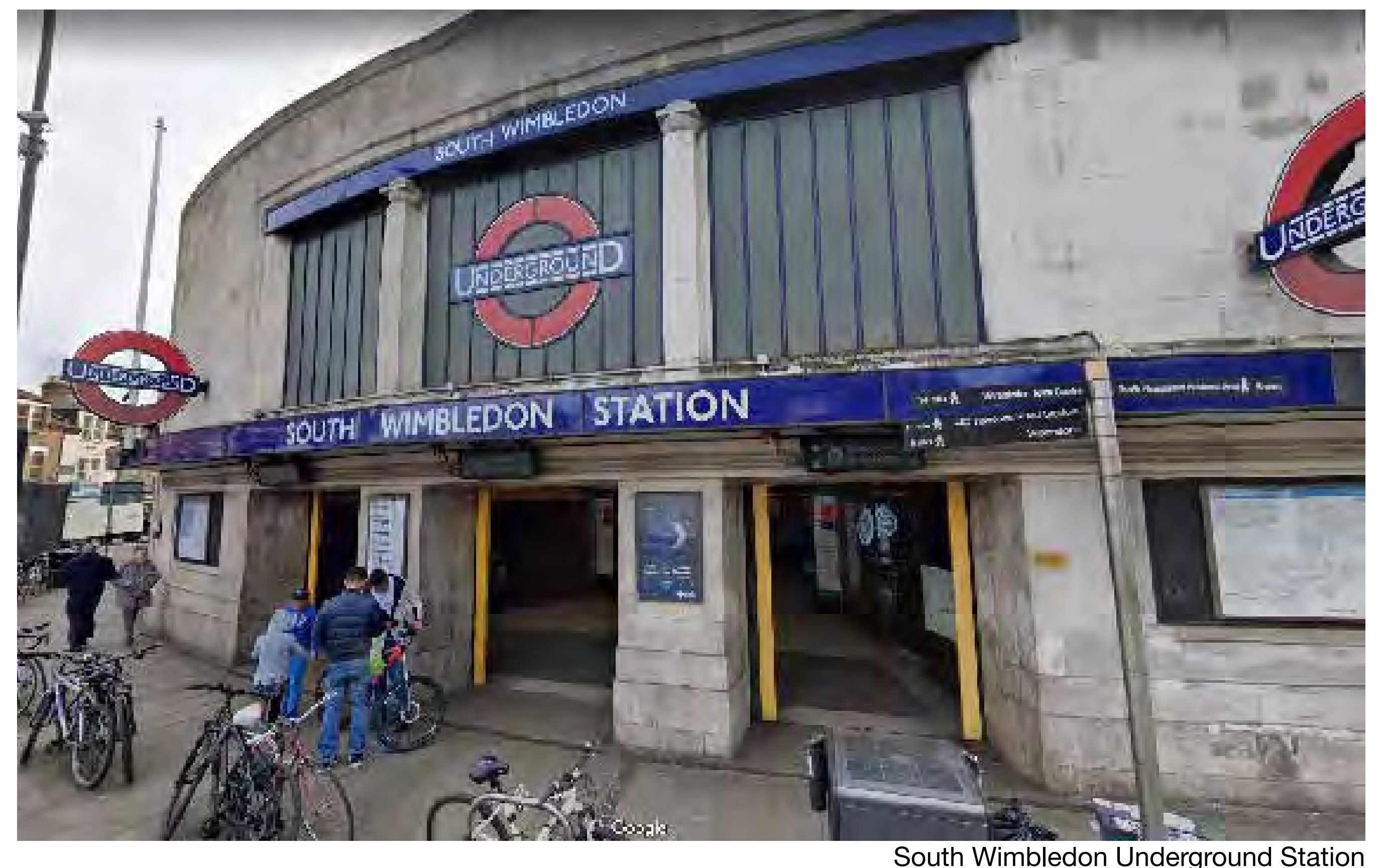
South Wimbledon Underground Station
